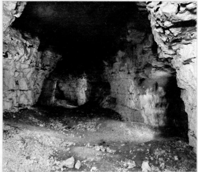
Hanover mine - This picture shows the shotcrete sprayed on the ceiling by Wimpey
